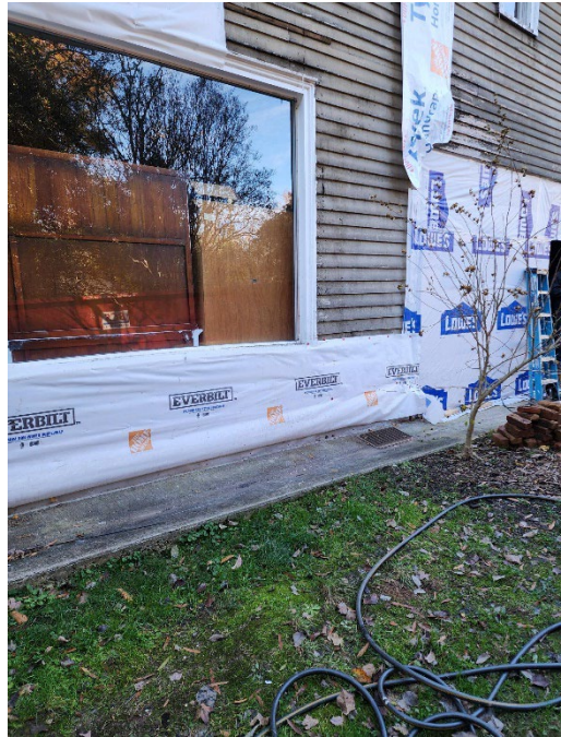
Plate glass window to be replaced with salvaged originals
